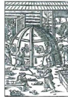
Antique glass melting furnace
