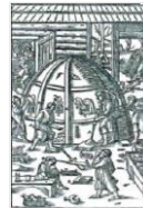
Antique glass melting furnace
