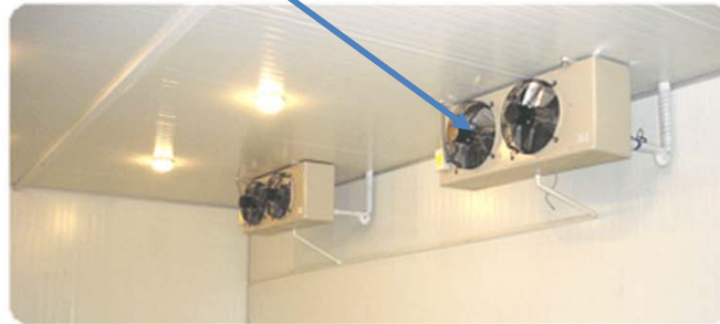
Cleanroom Cooling Coils
